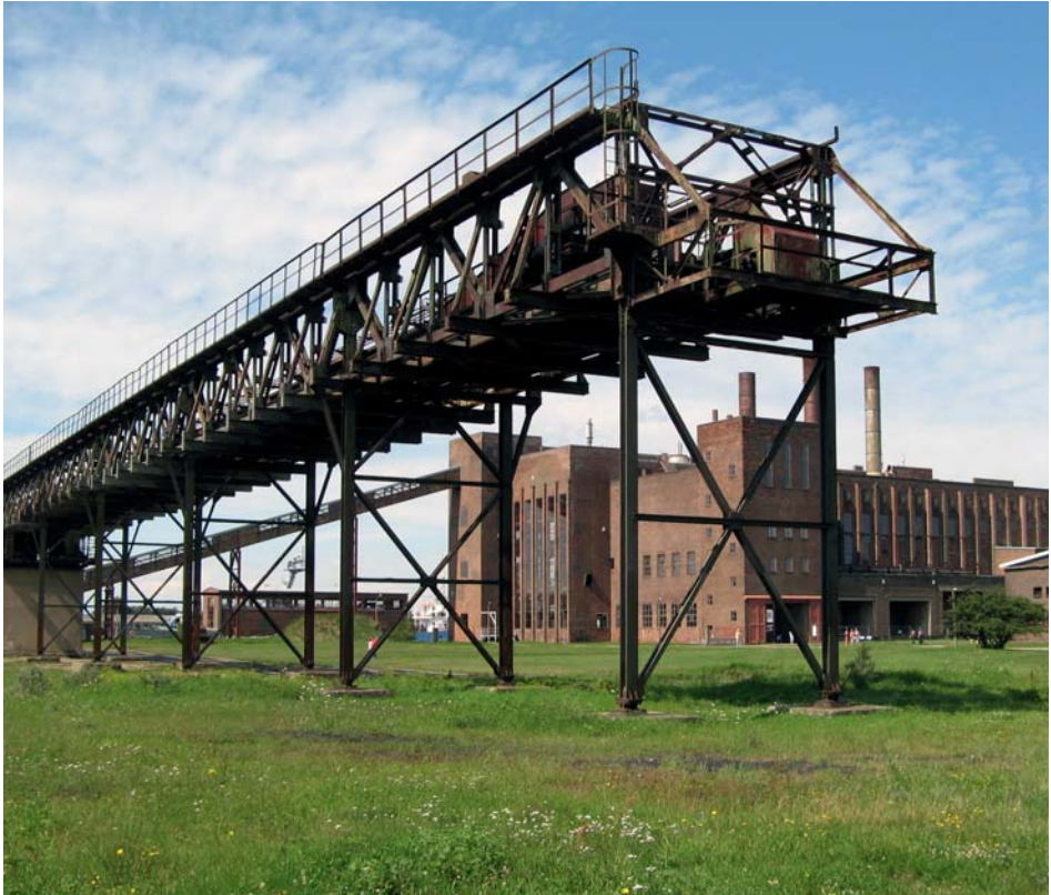
Coalbridge at powerstation of the former V2-rocket army testing site in Peenemünde, Usedom (Germany). Photo by Hans-Peter Balfanz.
