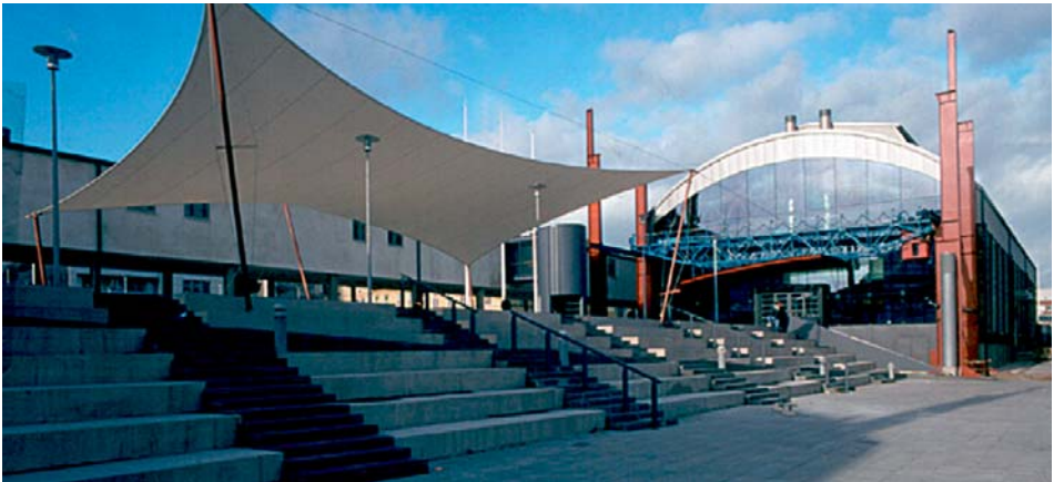
The old dockyard hall and rope factory in Turku was converted into spaces for the Turku Arts Academy in 1996. Photo by Hannu Matikka.
