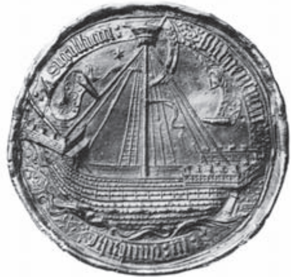
The seal of Gdańsk from 1400 represents the typical holk from the first half of the 15th century.
