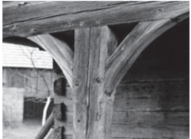
Zdrojno, detail of the arcade's construction.
