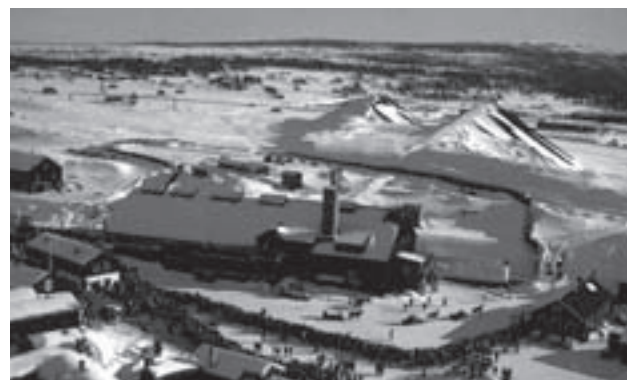
The smelting plant at Røros, seen here from the church tower.
