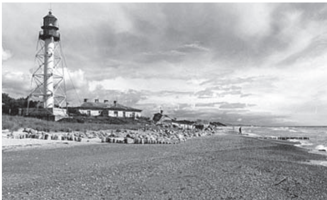
Pape Lighthouse (1910), situated Liepāja District, Rucava Parish, Pape. The 22.3 m high cylindrical tower is made of riveted steel sections framed in steel openwork. The tower is crowned with a small balcony and a light chamber with a weathervane above it. The illumination equipment has been modernised. The historical building complex includes a living house for the keeper, a machinery house, warehouse, and a cellar. Photo Andris Biedriņš.
