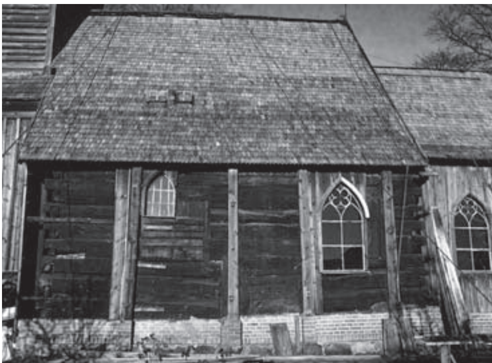
The church in Szczodrowo; type of corner joint made by carpenters. The church (its nave) was built in 15th century.
