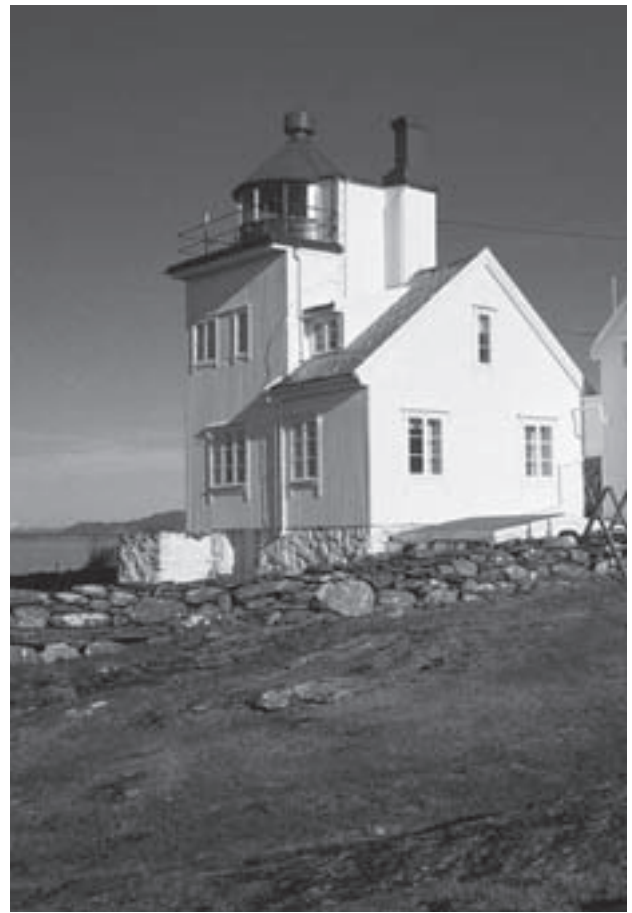
Tungenes built 1828. Decommissioned in 1984 and now used as a museum and cafe. Photo Kate Newland.
