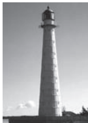
Tahkuna (Tackerort) lighthouse on the island Hiiumaa. Built in 1875 by British engineer Gordon, it is the highest cast-iron tower in Estonia.
