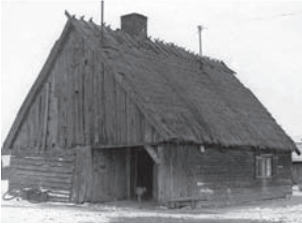
The house in Loryniec. The house with arcades; remodelled in 1930. We are going to show its original form at the museum. The walls are of horizontally set pine beams, dove-tailed at the corners.
