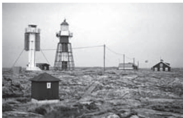
Måseskär lighthouse station on the Swedish west coast has a characteristic Heidenstam lighthouse. It is an example of a lighthouse run and taken care of by a private foundation.
