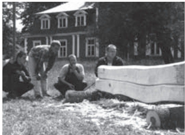
Carpenters at work at Ungurmuiža manor house in Latvia.
