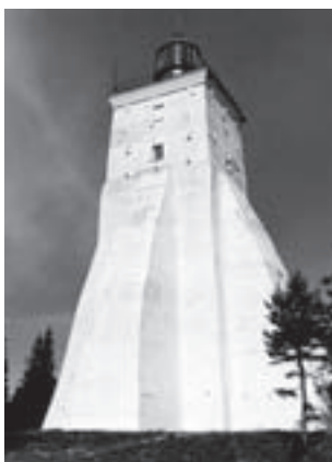
Kõpu (Dagerort) lighthouse on the island Hiiumaa. Built in 1531, rebuilt in 1810, 1845 and 1990. The oldest lighthouse still in use in the Baltic Sea region.
