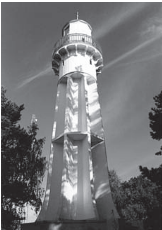
Mersrags Lighthouse (1875), situated in Talsi District, Mersrags Parish. It is a freestanding cylindrical riveted iron tower 18.5 m in height. After it was destroyed in World War I, its lower part was embedded in concrete and fixed in reinforced concrete. In the upper part of the tower, there is an enveloping steel balcony supported by steel cantilevers. The light chamber is crowned with a domed roof ending in a decorative spherical projection and a weathervane. Photo Andris Biedriņš.
