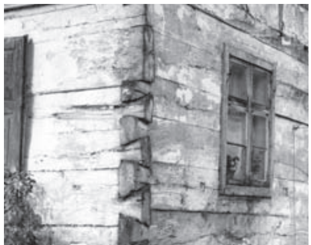
Luzino, detail of corner construction (Quoin).
