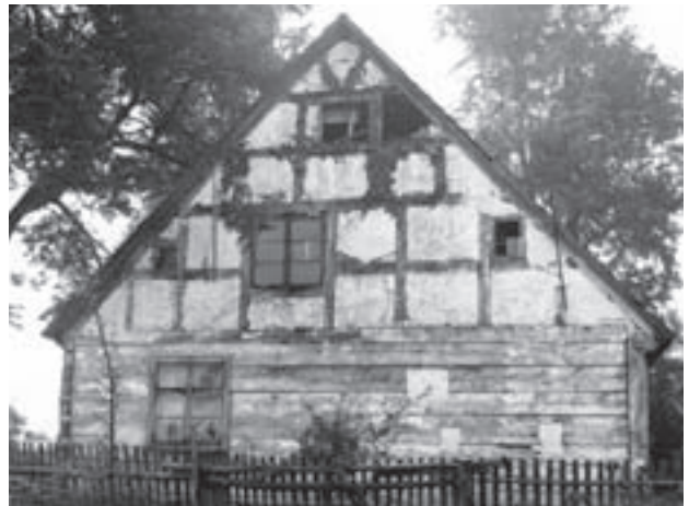
Luzino, gable-end frame work wall.
