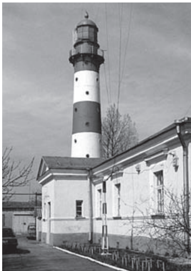
Liepāja Lighthouse (1868), situated in Liepāja. The conical tower of the lighthouse 29 m in height was assembled from 30 mm thick cast iron segments joined together with screws. Inside the tower, there is a cast iron winding staircase. It is the only lighthouse tower in Latvia made of cast iron segment constructions. The author of the project, as well as the supplier of illumination devices was an English company: Chance Brothers Near Birmingham. The sections of the lighthouse shot during World War I were cast anew in the workshops of Liepāja Naval Port. The housing complex of the lighthouse includes a living house for keeper and machine house, both united under one roof. Photo Andris Biedriņš.
