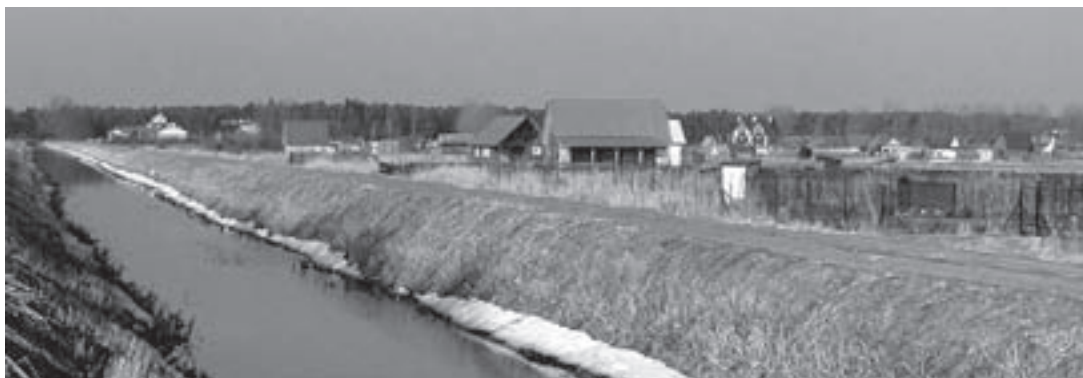
The new sub-standard building on the land adjacent to the seashore in the region of Karwieńskie Błota.
