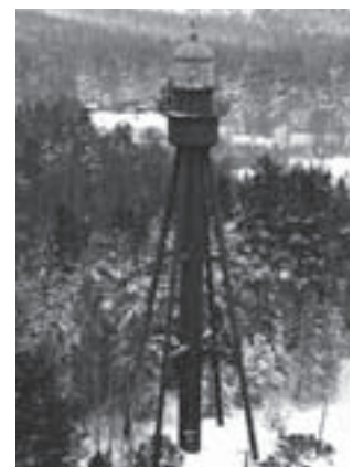
Ruhnu (Runö) lighthouse on island Ruhnu in the Gulf of Riga. Built in 1877, its iron components were shipped from Le Havre. Reconstructed in 1937.
