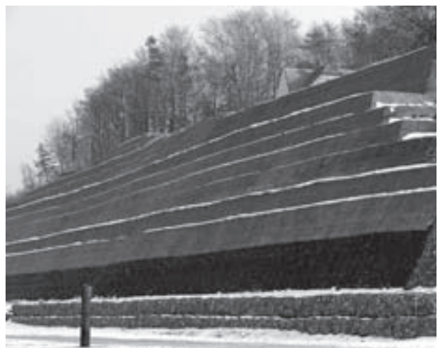
The reinforcement construction protecting the cliff at Jastrzębia Góra has completely ruined its natural landscape.
