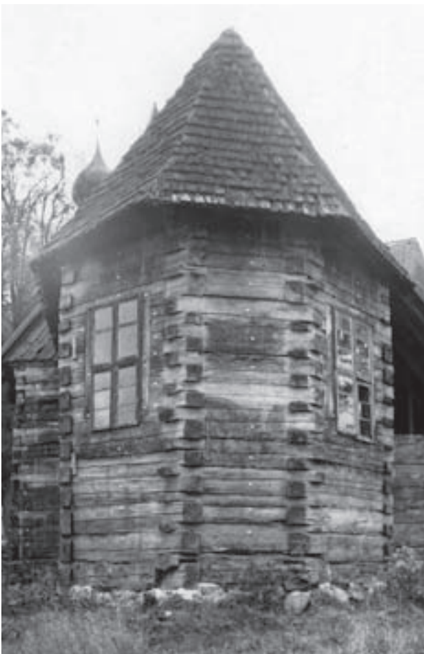
The church in Swornegacie. The church before dismantling; without exterior boarding.
