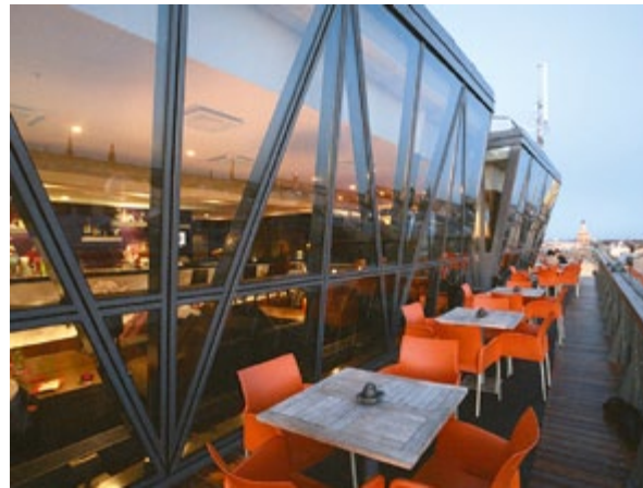
Rebuilding of the block surrounded by Antonijas, Dzirnāvu and Zaļā streets. © "Arhis"
