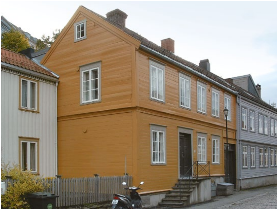
The log house has been upgraded by better insulation and heating with bio fuels and utilizing solar energy. Bakklandet, Trondheim, Norway.
