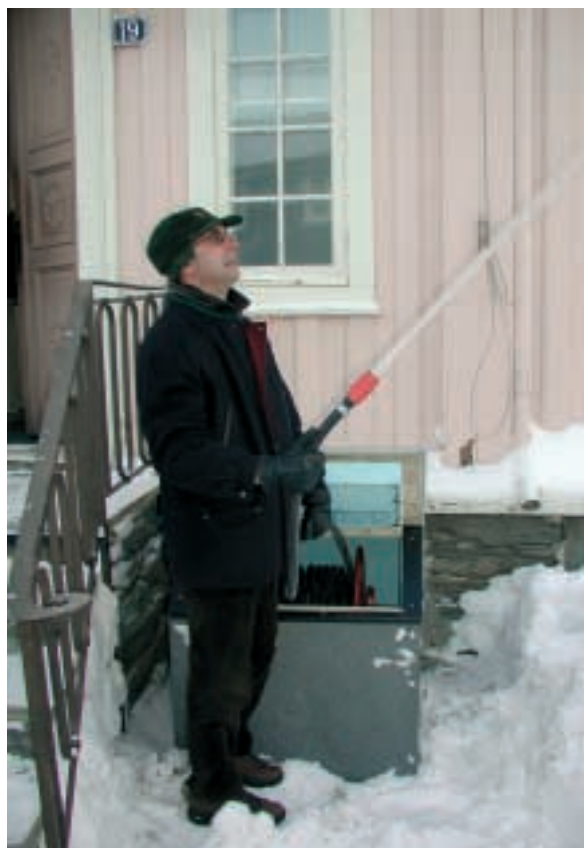
Plastic fire hoses are easier to use than the ones made of cloth because it is not necessary to pull it out full length.
