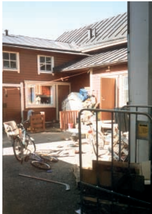
There is still too much combustible material in some of the courtyards in Rauma.
