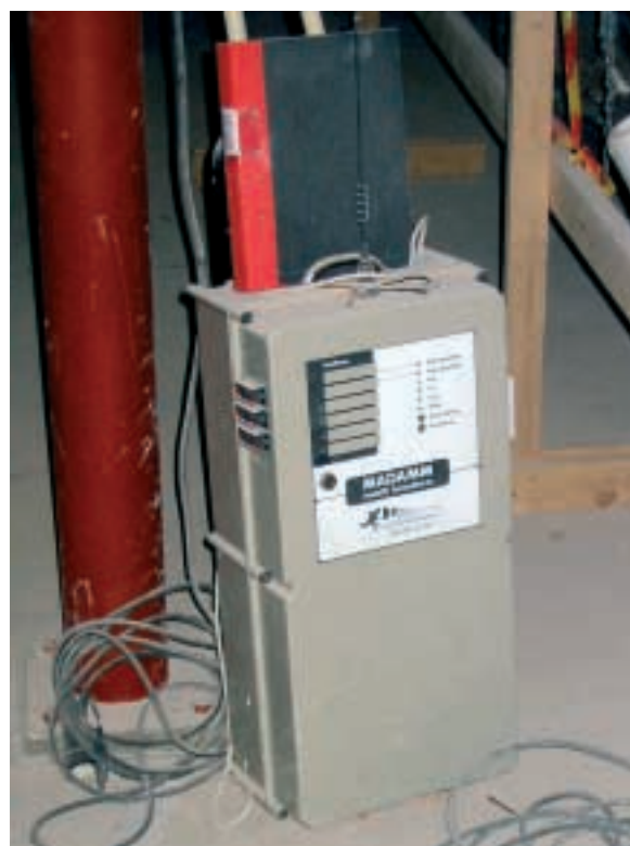
“MADAMM” a movable air sampling fire detector.
