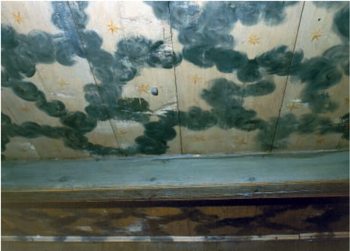
The only visible part in air sampling systems is the tiny end of a plastic pipe – if it is possible to hide the main pipes in such places as the attic above.
