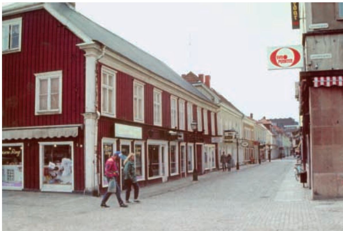
The block in Jönköping before the fire.
