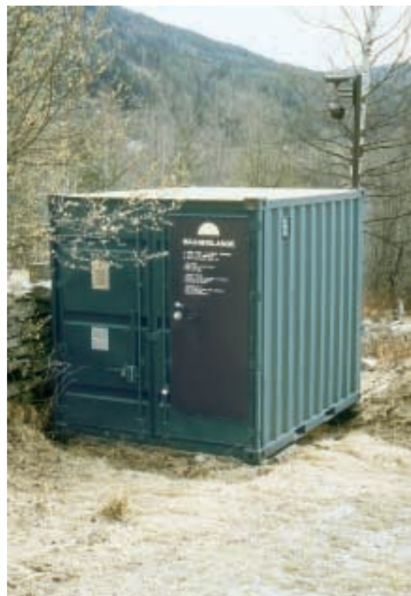
A mini fire station in Norway.
