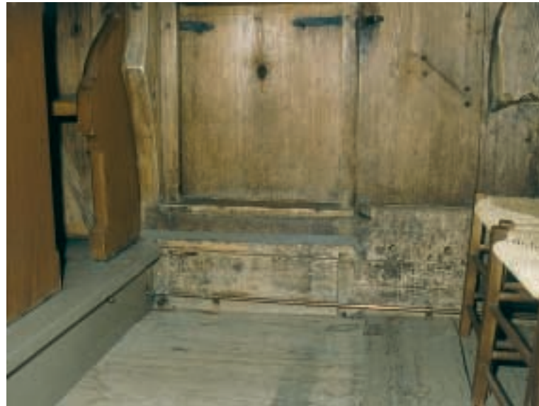
Copper sprinkler pipes match well with aged wood.
