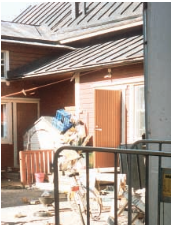
It is easy for an arsonist to set fire to an open bin full of rubbish in the vicinity of an historic building.
