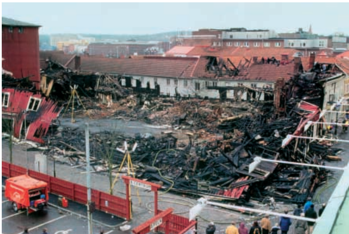
The block in Jönköping after the fire.
