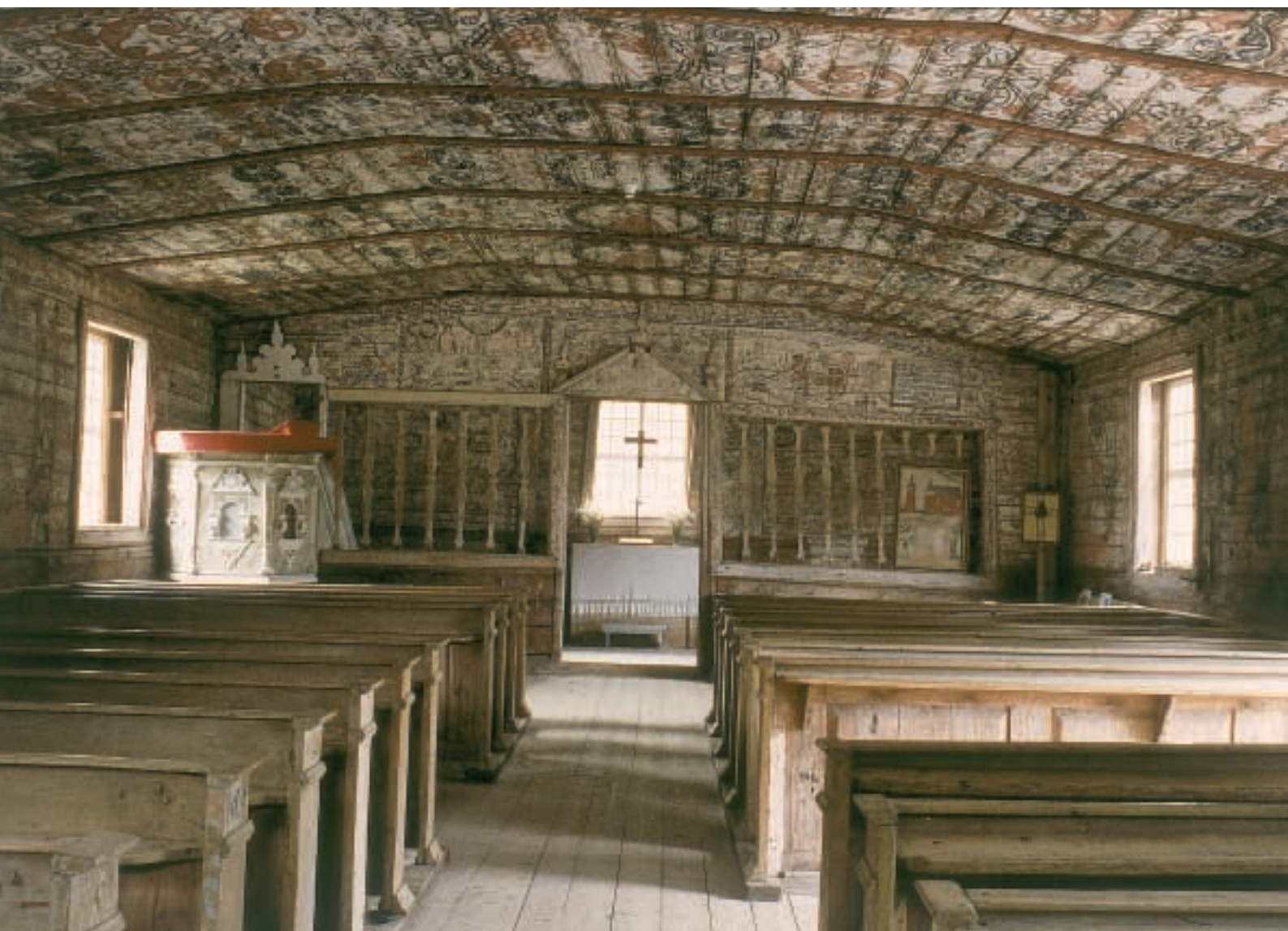
Many indoor paints such as sensitive glue-based paint do not stand the amount of water that traditional sprinkler systems need, so a water mist system is more suitable for this kind of interior. (Pyhämaa Church)
