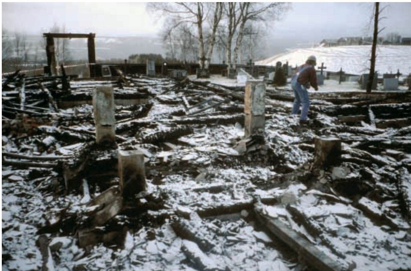
The starting point for investigations after a fire can be like this (Innset church, Norway).
