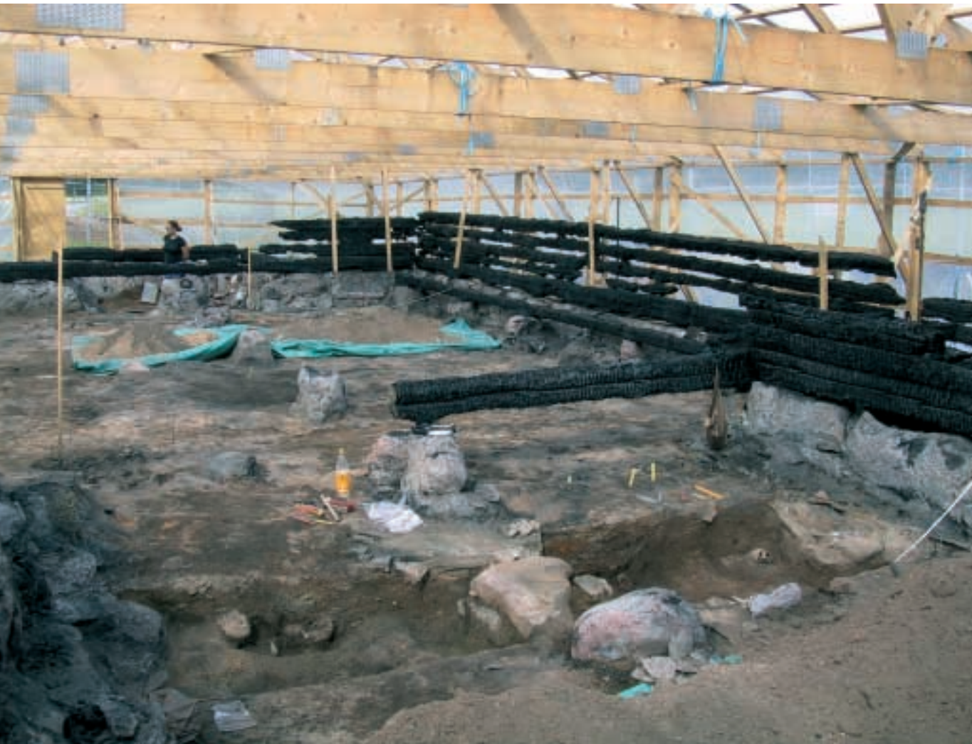
Protective construction was built to cover the remains of Södra Råda.
