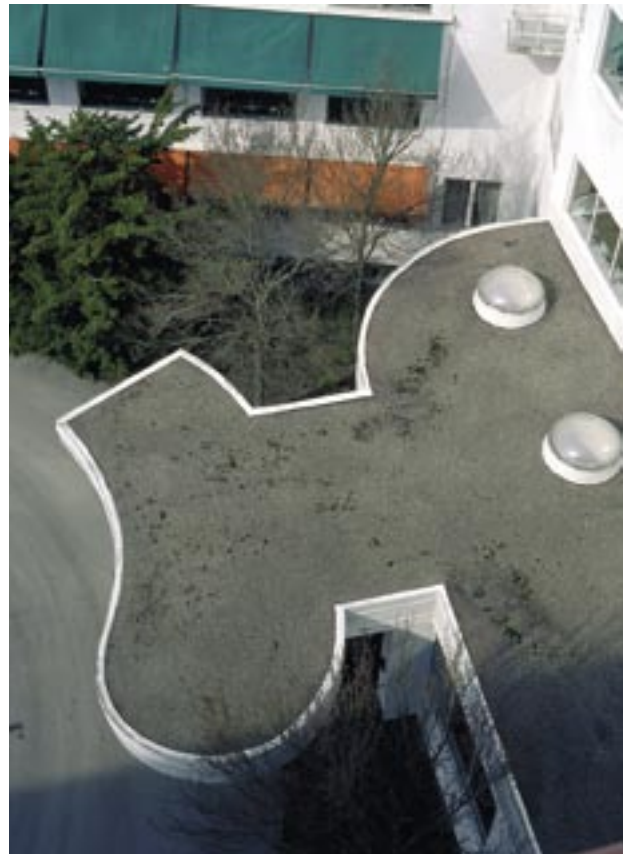
Fig. 61. The main entrance canopy.
