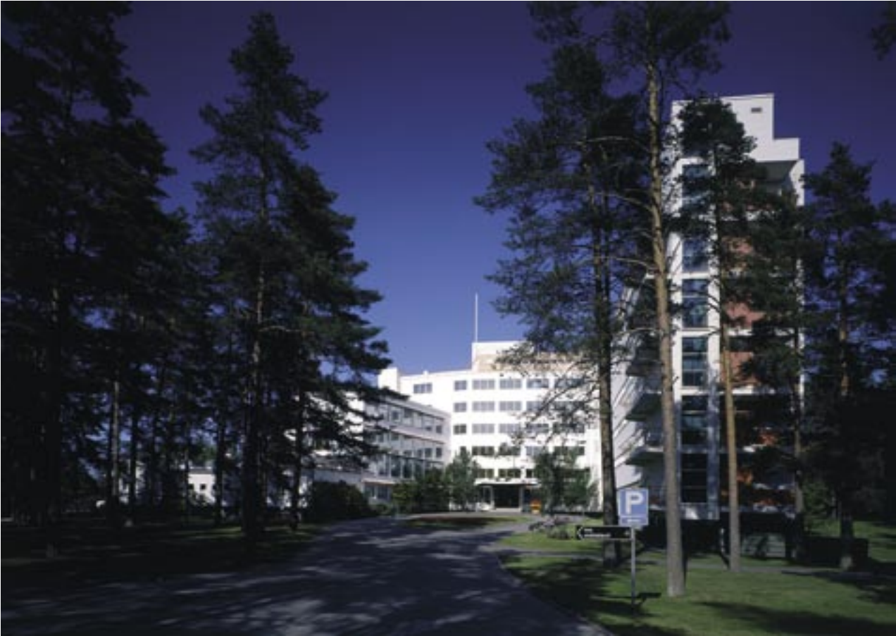
Fig. 11. A view towards the main entrance: on the left is the wing containing the communal spaces, on the right the end facade of the patients' wing.
