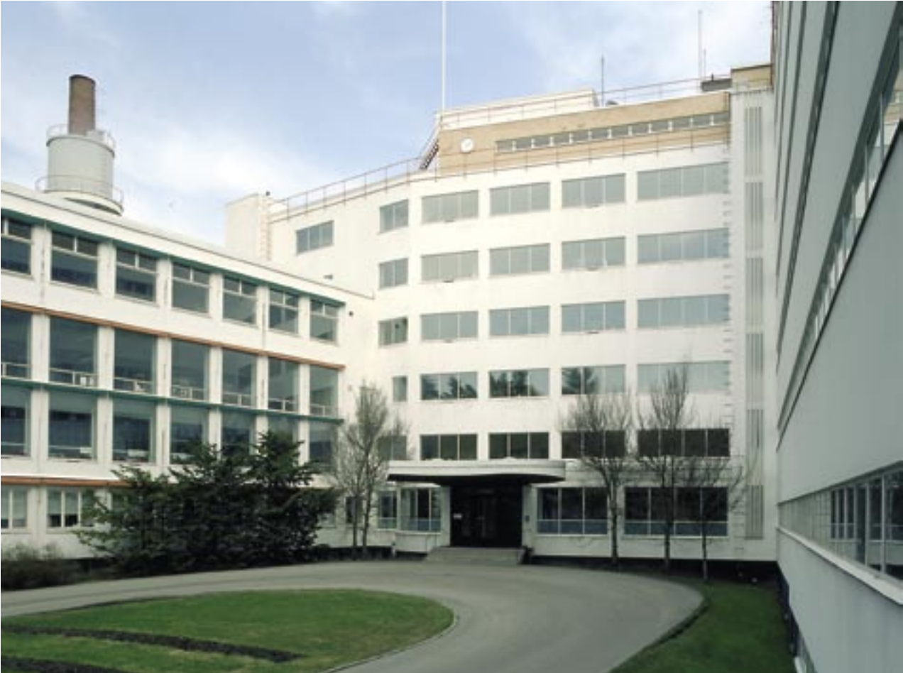
Fig. 30. The main entrance courtyard of the hospital.
