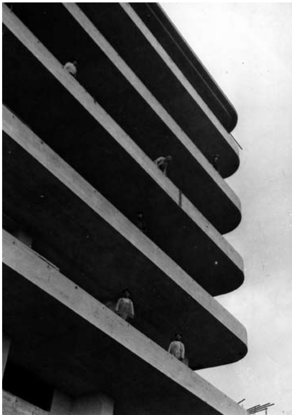
Fig. 24. Building workers on the patients' sun balconies.
