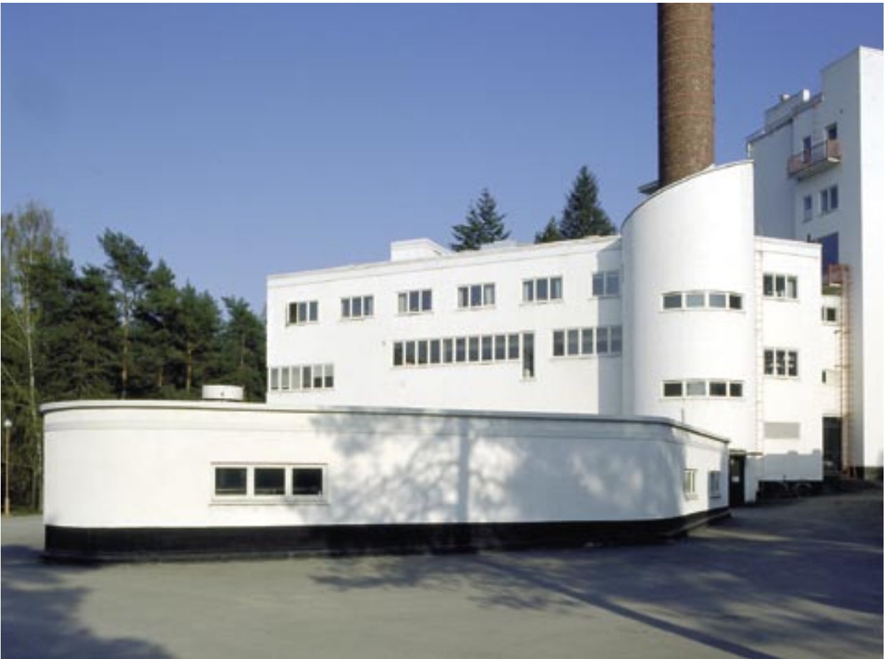
Fig. 15. The kitchen and maintenance wing. The building in the foreground originally housed a heating plant.
