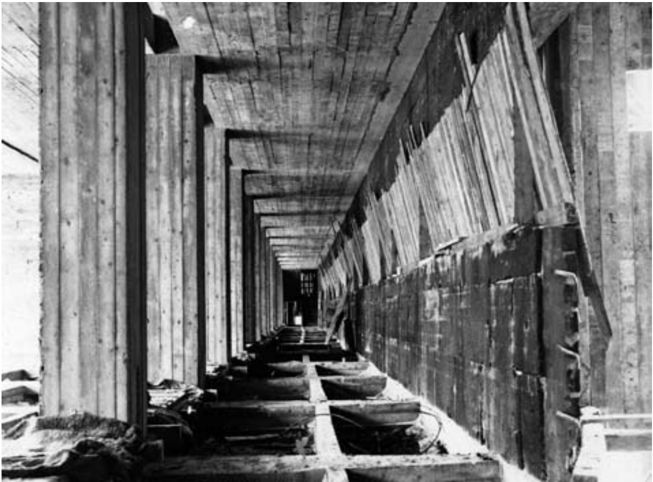
Fig. 23. The concrete structure of the corridor of the patients' wing.
