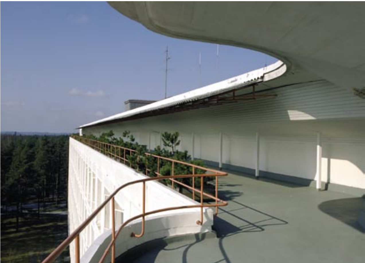
Fig. 8. The concrete overhang of the rooftop sun deck.
