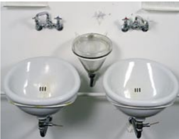
Fig. 33. The 'non-splash' washbasins and spittoons.
